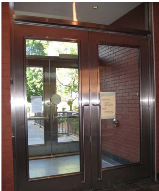
View of City Hall/Library automated opening doors
